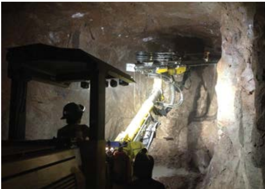
Left – Drill rig preparing a development heading for blasting
